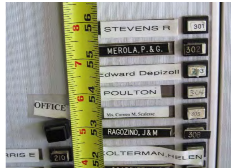
Original intercom panel at main building entry – Note some buttons exceed handicap accessibility reach limits
