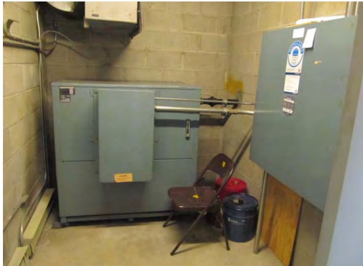
Original hydro-mechanical pump unit and controller/dispatcher for elevator
