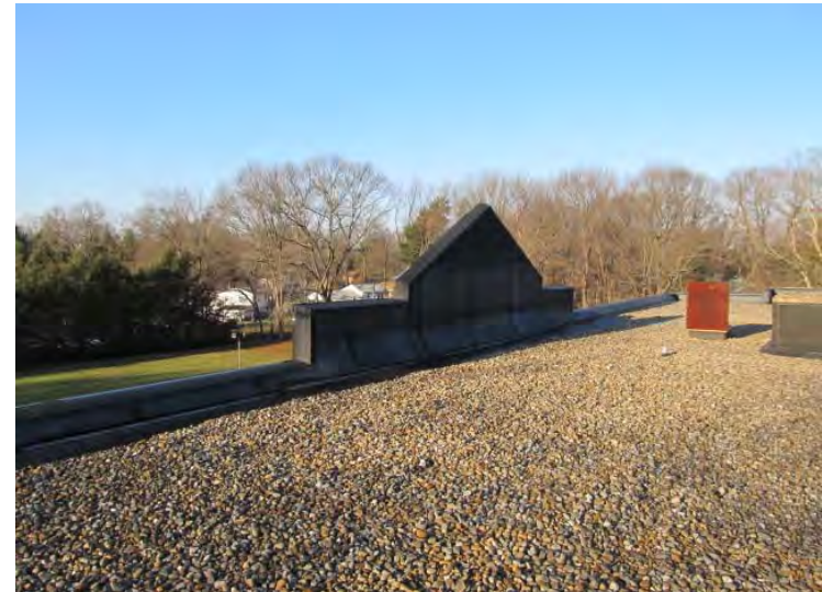
Water infiltration issues and past repairs reported with regards to ballasted membrane roof covering
