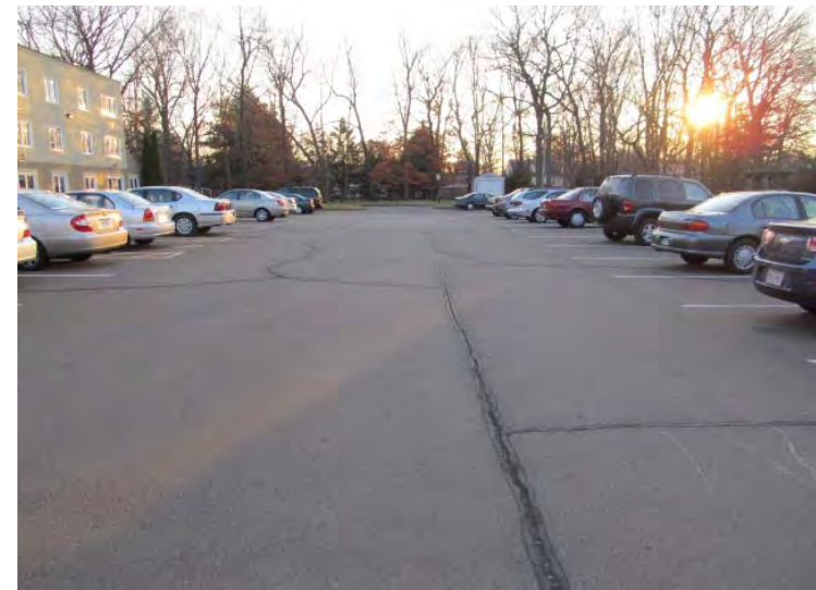
Asphalt paving in generally good condition – Routine surface maintenance needed in near-term
