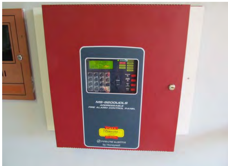
No problems related to newer, fully addressable, fire alarm control panel were observed or reported
