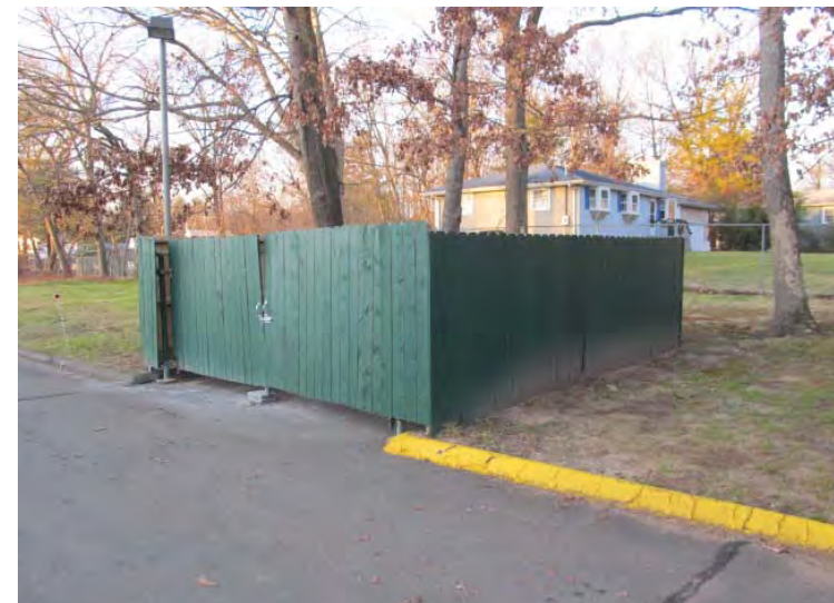
No significant wear or damage noted at wood stockade dumpster enclosure
