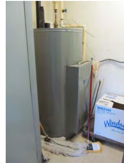
Original electric domestic hot water tank that serves interior common areas
